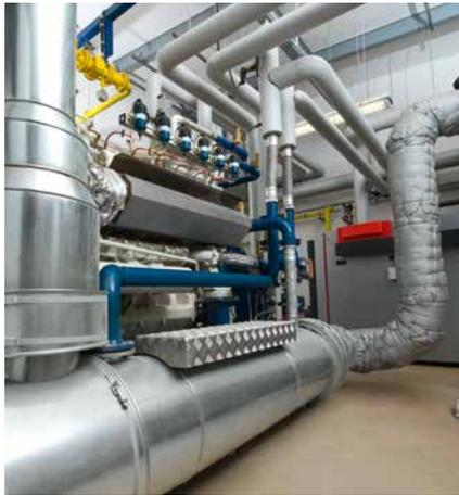
Exhaust gas catalytic converters reduce the polluting emissions which are produced when the engine is in operation. They reduce poisonous carbon monoxide (co), hydrocarbons (hc), aldehyde (odour), nitrogen oxide (nox) as well as particles which are hazardous to health and already reach high conversion rates at low temperatures.
